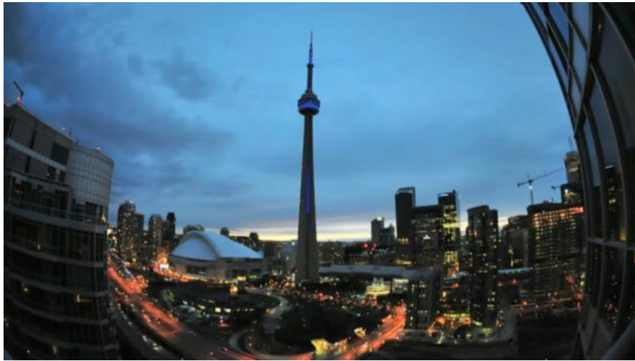
"Fig. 1. E-TOWER (tower view), Oct 2, 2010, Dave Colangelo and Patricio Davila, Installation.
