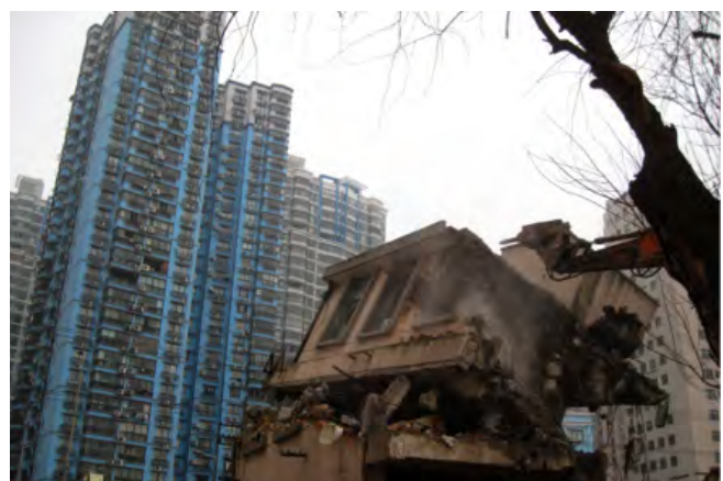
Fig. 12. Demolition in Shanghai, 2010, Bert van Dijk, photograph, Creative Commons license.
