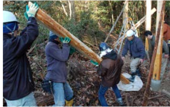
Figure 5, erecting the pillars
