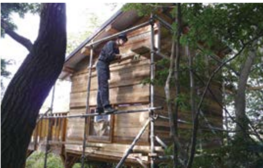
Figure 9, building the walls
