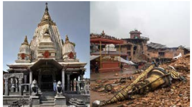
Figure 1: The historic area of Bungamati (Rato Machendranath) – before and after April 2015 Earthquake. (Photo credit: left Mauro/Ornella, right Omar Havana)
